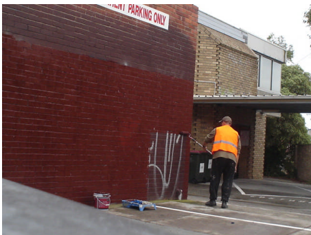
1) Removal takes place
